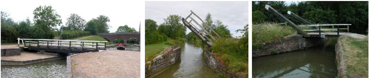
Image 4-6 - counterweight and swing bridge designs commonly seen on canal network (© Mike Todd, Geograph CC)
